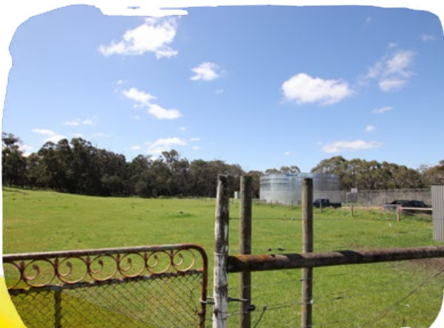
Left: Sewerage treatment facility at Maryknoll TC Right: Members of the Corporate Services Team
